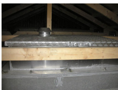
Nedgang ny rentvandstank Under taget
